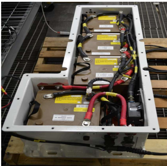
Figure 6 Battery Enclosure with top removed
